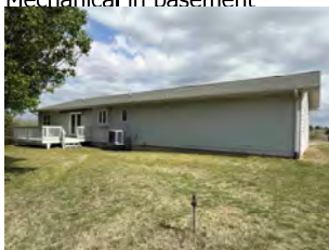
Back Of Structure
