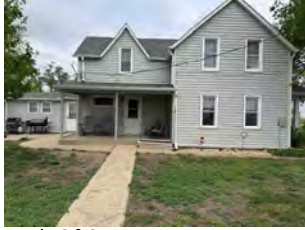
Back Of Structure
