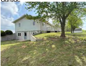
Back Of Structure
