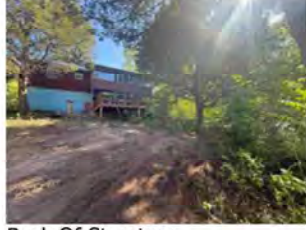
Back Of Structure
