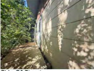
Side Of Structure
