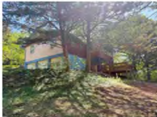
Back Of Structure
